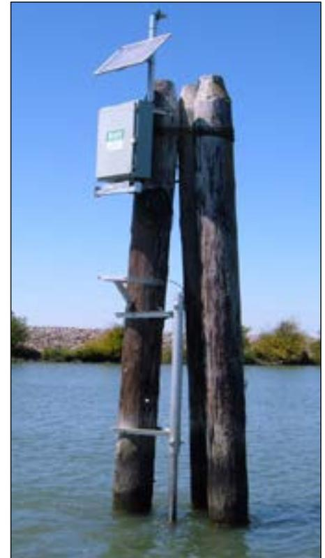
*Flow station on channel piling.
